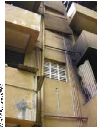
Blackened walls due to lack of proper chimneys and exhaust system to absorb the excessive smoke generated by firewood which is used traditionally for cooking.
