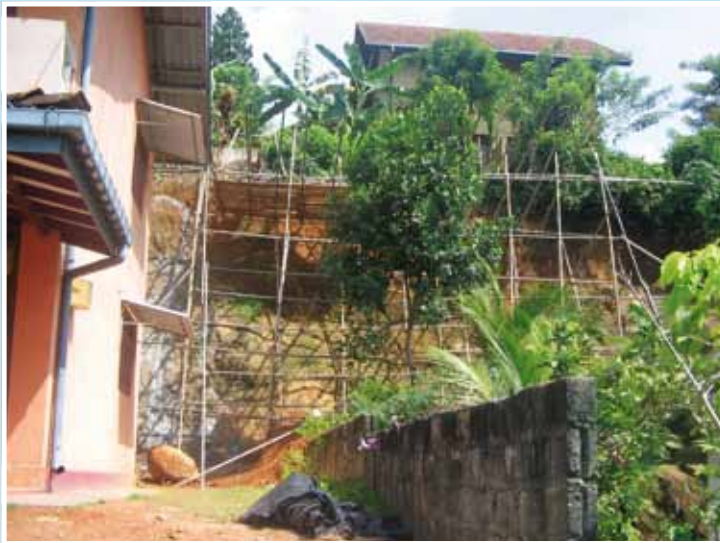
Retaining walls being reinforced to avoid housing from getting damaged or collapsing.
